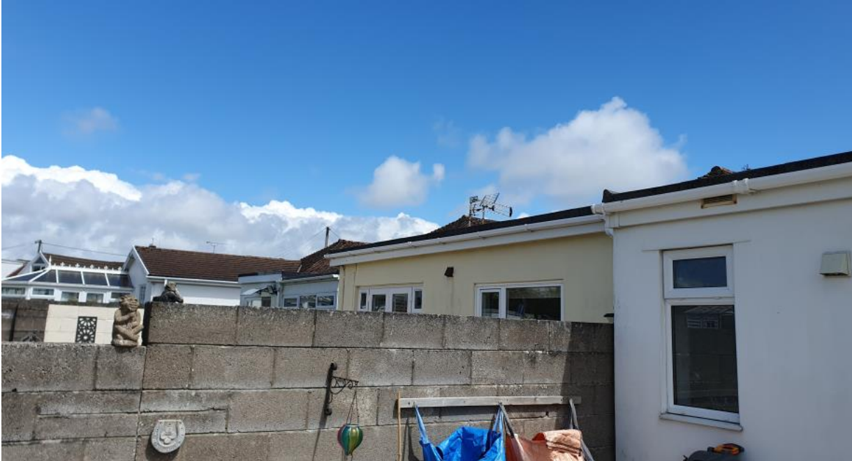
Figure 5 - Image showing other extensions
